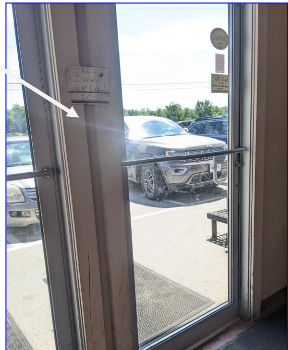
A sign at Allen Brothers in Westminster marks the height of Flood waters in the wake of Tropical Storm Irene in 2011.
