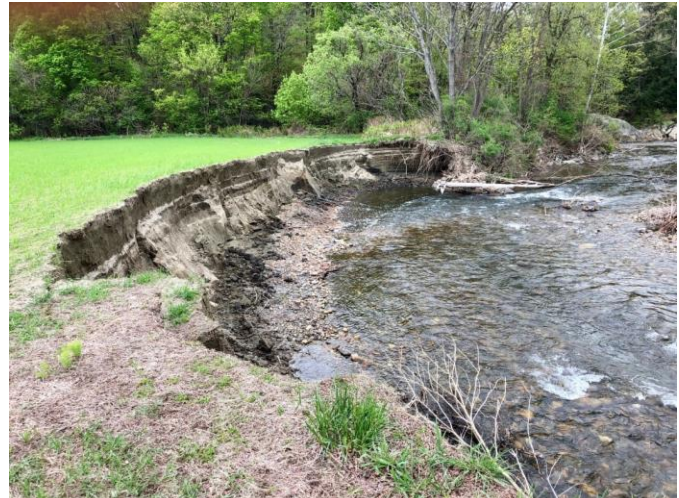
Fluvial erosion site along the Saxtons River at the Basin Farm. – Photo courtesy of Peter Bergstrom.
